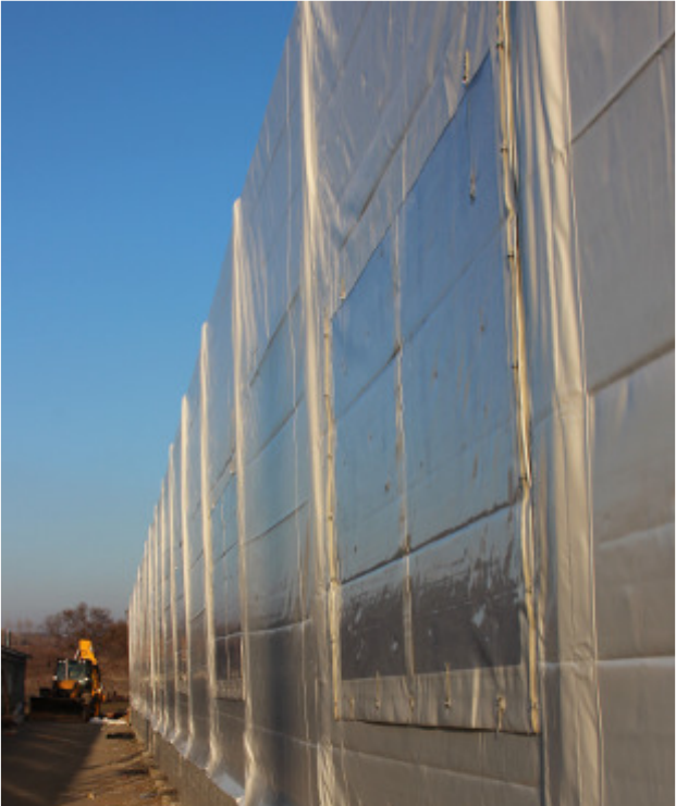
Ventilating valves from transparent fabric, an inside layer from the PVC mesh
