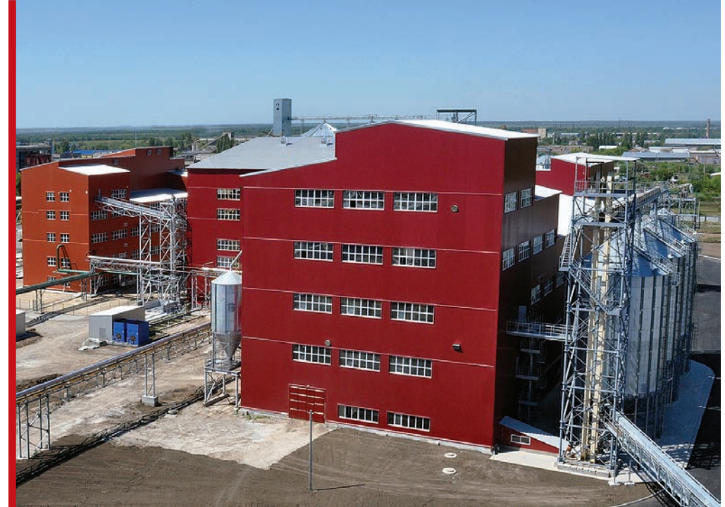
05. | COMPLETED PLANT JULY 2012
